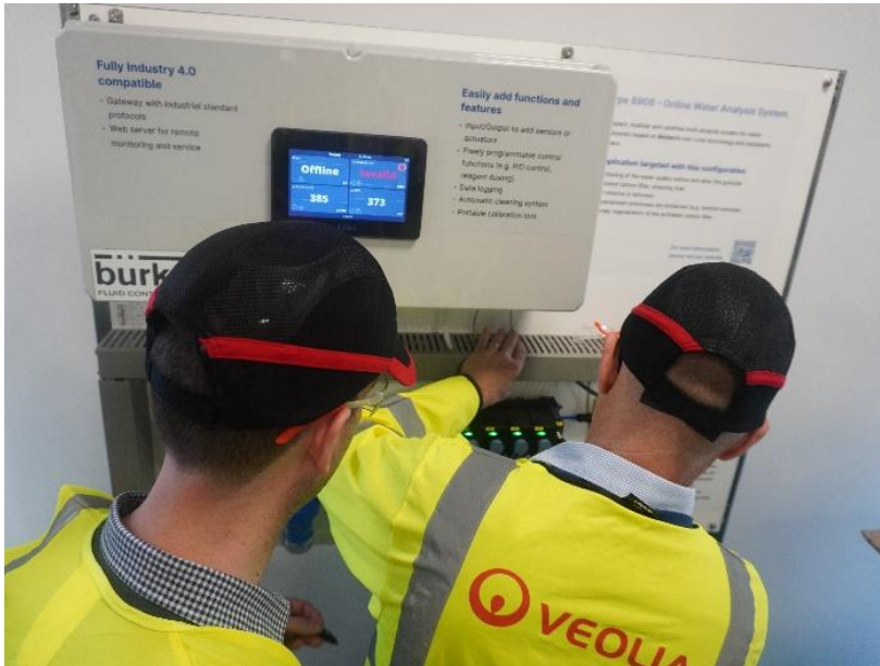
Image 1: Installation of the compact Online Water Analysis System was a simple process.
